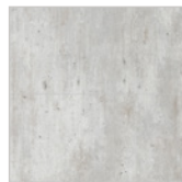
Cracked Cement, pictured left M6030
